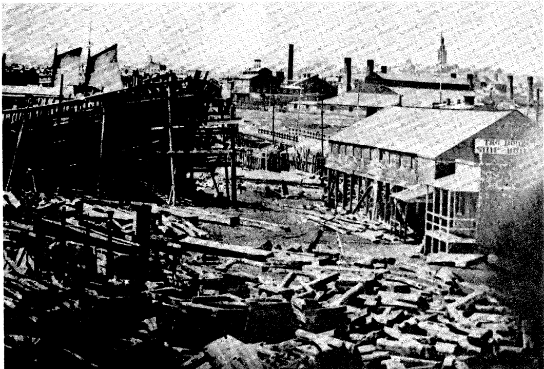
Thomas Booz and Brother Shipyard, Canton, about 1875. Steambox at center for softening planks, mold loft at right.
