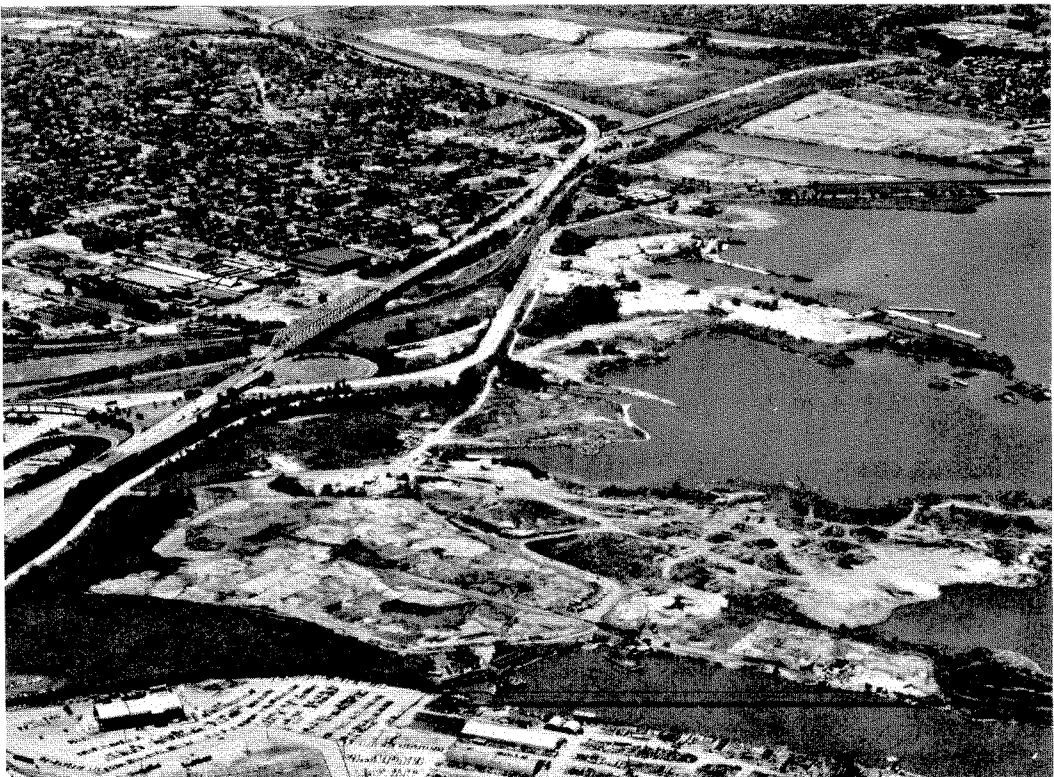
Masonville, Southwest Branch of the Patapsco River
