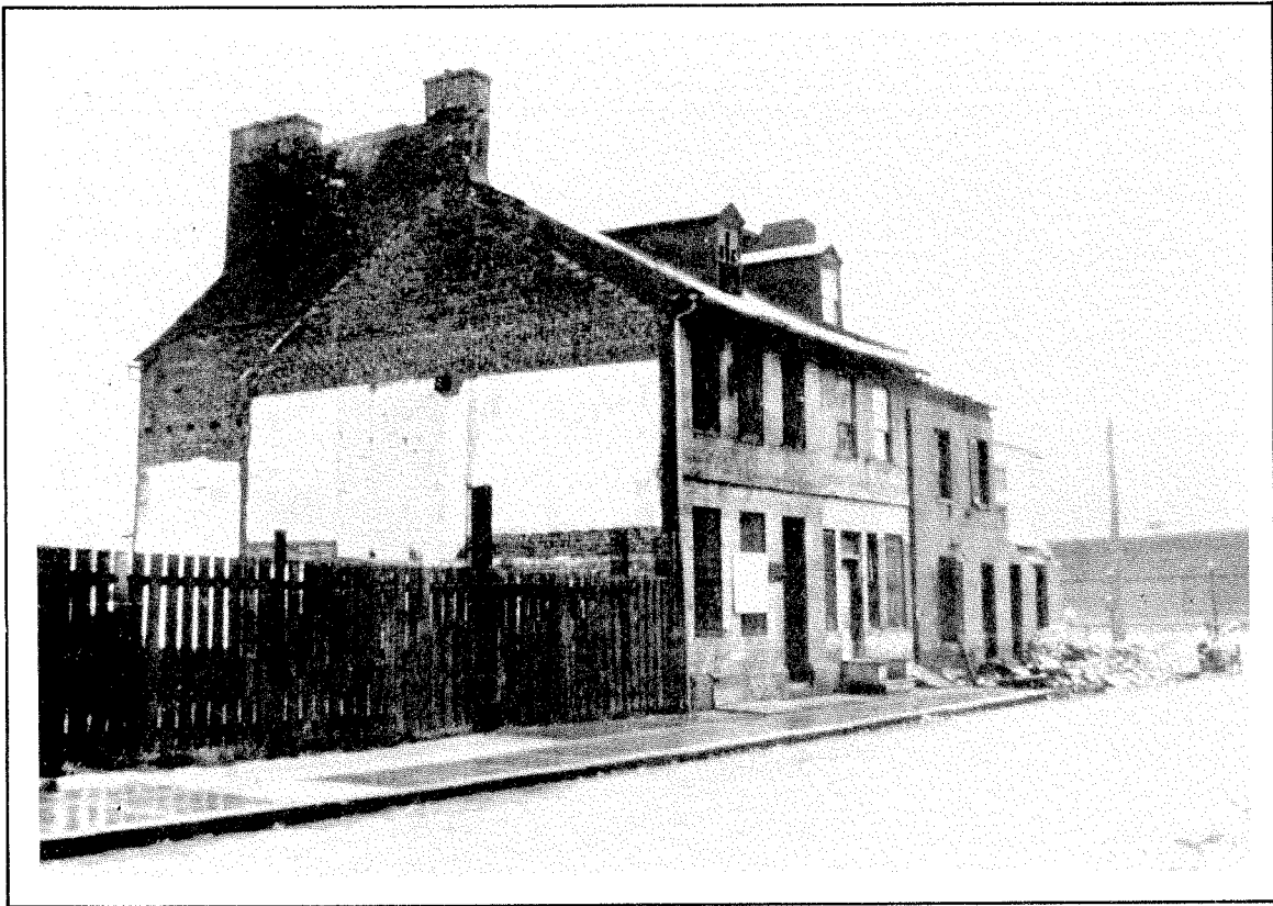
Houses being torn down Many of the original homes were razed in the middle 1930's for commercial purposes
