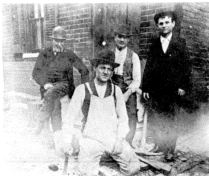
Restoring brick sidewalks, 1890's
